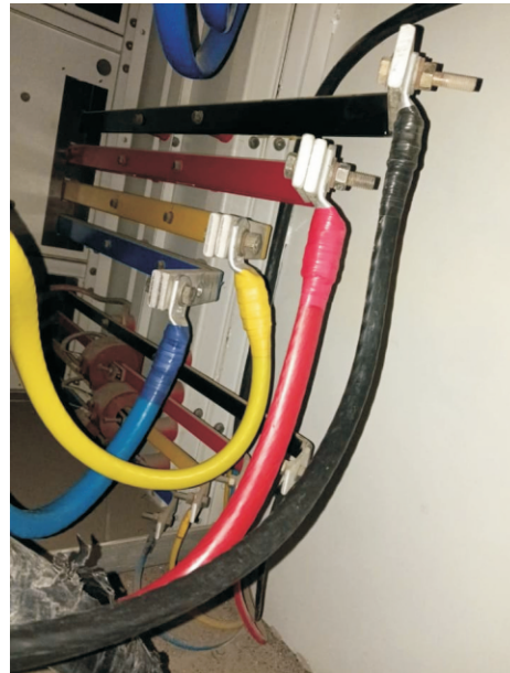
Cable Termination Installation
