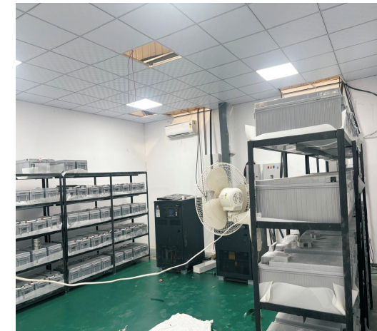
UPS & Battery Installation
