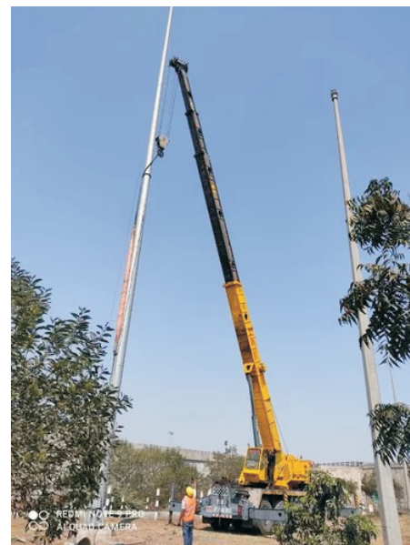
High Mast Installation
