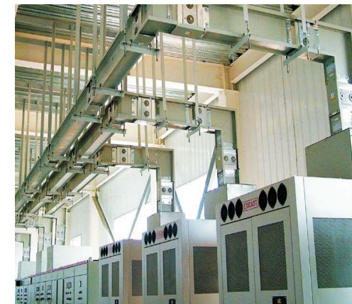
Bus Duct Installation
