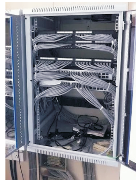
CCTV Rack Installation
