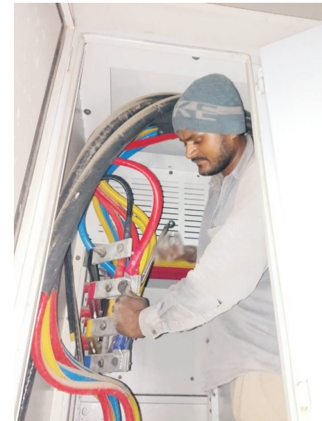
Panel Termination Installation
